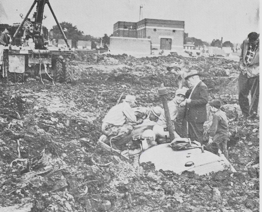
Residents of the area north of Frenchmen's Bay, Ont., knew this could happen and it finally did. Spreading sand on a muddy section of land, a bulldozer began to sink when it was attached to it and heavy trucks tried to pull it out, but the machine just continued to sink.
