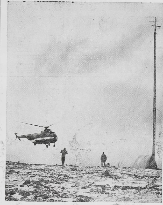
FROM A ROCKY HILLTOP rises a radio mast where a detection station of the Mid-Canada early warning line will be erected. The Sikorski helicopter is flying in an auxiliary power unit for the radio. RCAF helicopters have been flying between lakeside camps and detection sites on the top of hills. (National Defence Photo)
